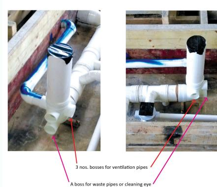
According to the regulations of Building Department, it is essential to use a standard fitting - Multipurpose High Vent Elbow to ensure the ventilation pipes being higher than the soil waste pipes in sunken. In order to have a greater flexibility, three nos. of bosses with different directions are equipped. 2 nos. of plugs are included for an elbow to clog the bosses. Besides, a lowest waste boss can be used as a cleaning eye or connection for other waste pipes.
